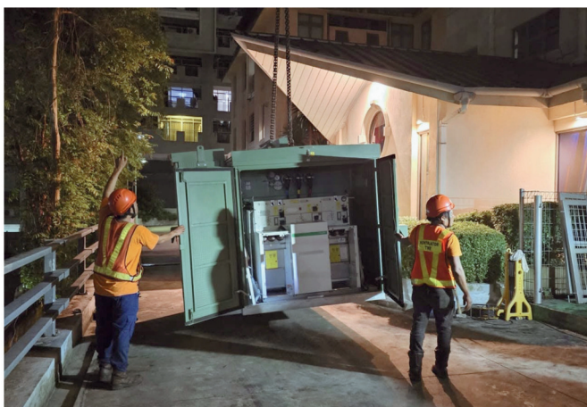
New Substation Put Into Position
